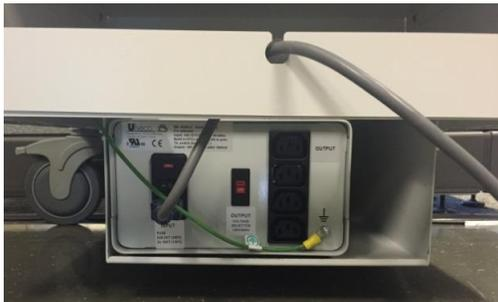
Connect the main AC Power Cord to the Isolation Transformer AC inlet as shown.
